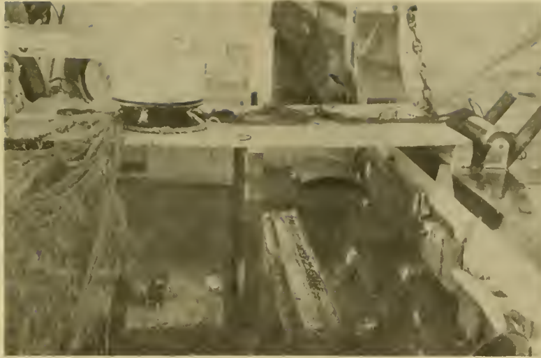
FIGURE 8 - ROLLERS AND TABLE USED IN HAULING THE GILL NETS.
