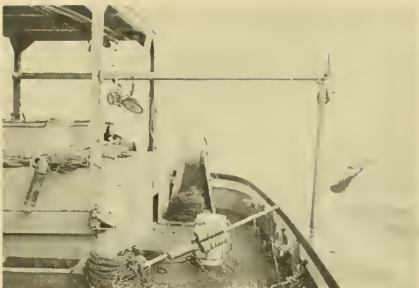
FIGURE 42 - GROUND LONG-LINE GEAR READY TO BE SET FROM THE STERN OF THE COBB . THE GEAR PAYS OUT OVER THE METAL CHUTE AS THE VESSEL RUNS AHEAD.
